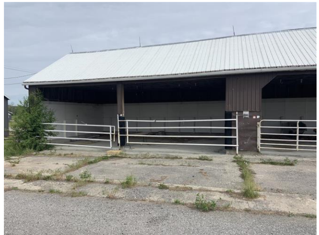
Photo 10: Existing conditions of IAGM1 community showing the agricultural building #35.
